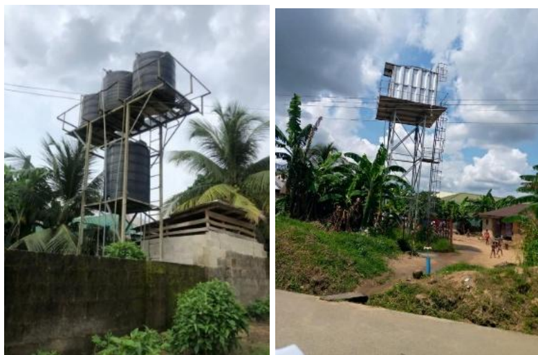
Plate 1: Borehole with Overhead Tanks for Water Supply in Adiabo Ikot Mbo Otu
