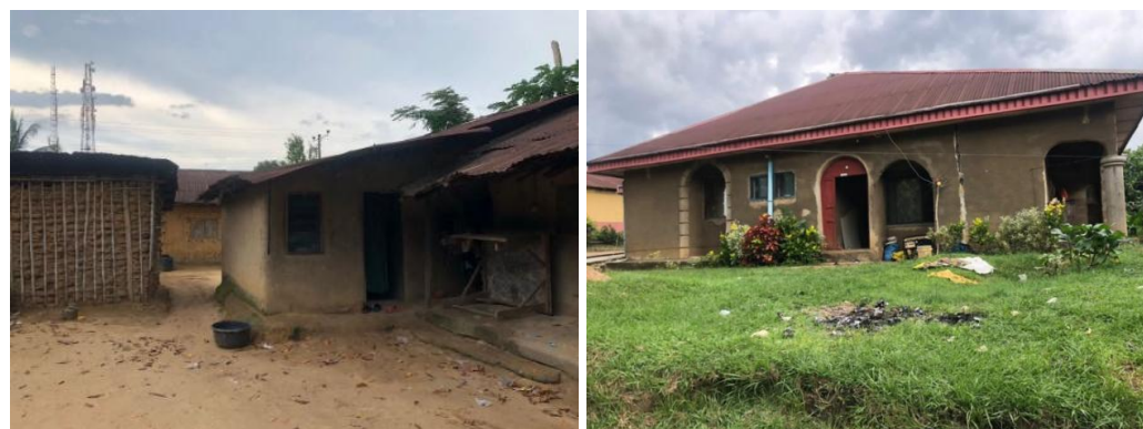
Plate 2: Building Materials Used in the Study Area (left, mud wall and right, cement wall)
