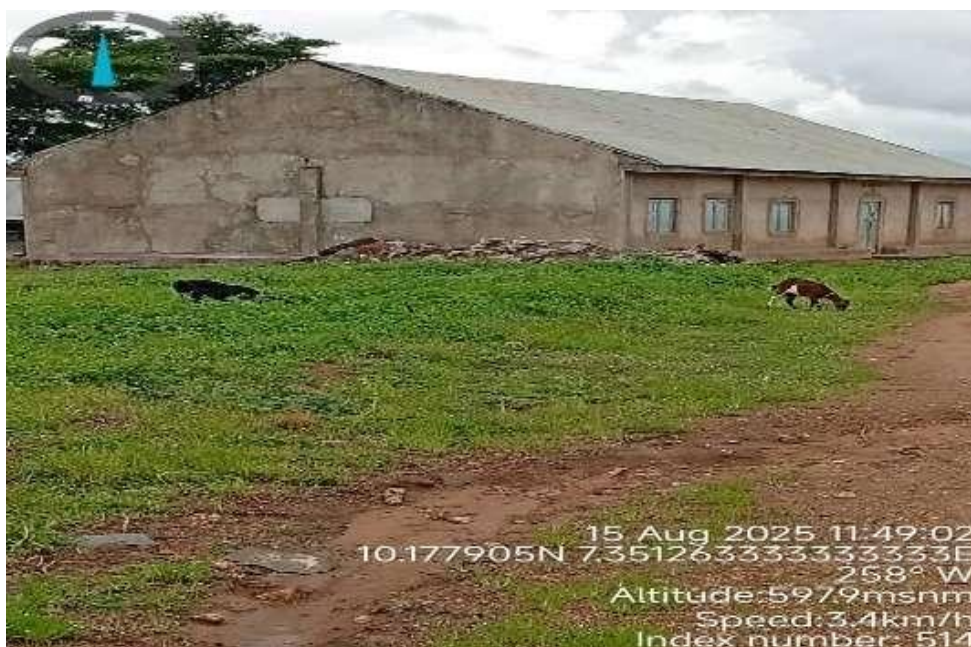
Plate 4.8 Community Church at sabon birnin Kasarami
