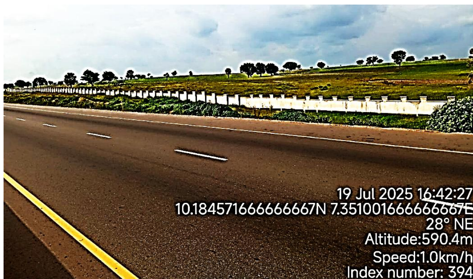
Plate 4.7: Abuja – Kaduna – Zaria expressway, adjacent to the AIH SAPZ site at Daki - Takwas
