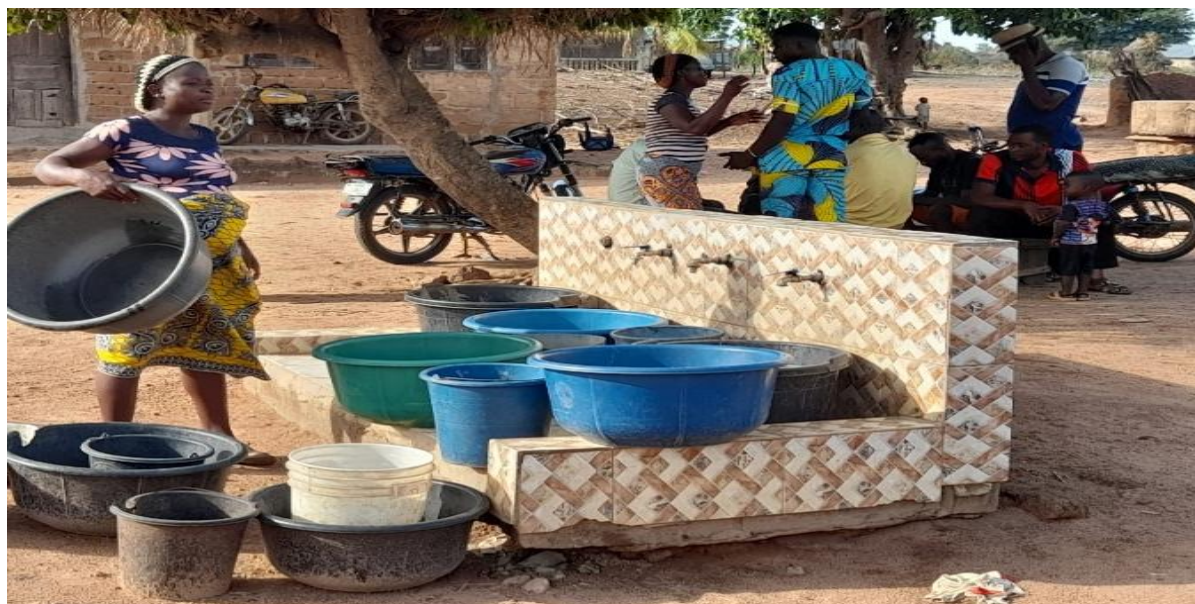
Plate 4.38::Community Borehole as captured in Daki Takwas
