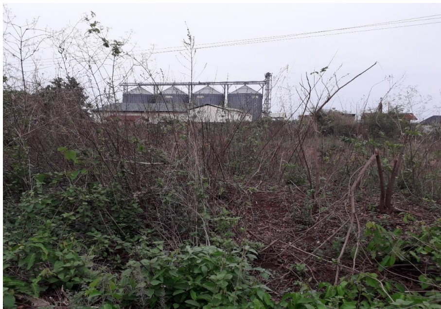
Figure 3.17: Silos constructed within the facility for storing and preserving grains
