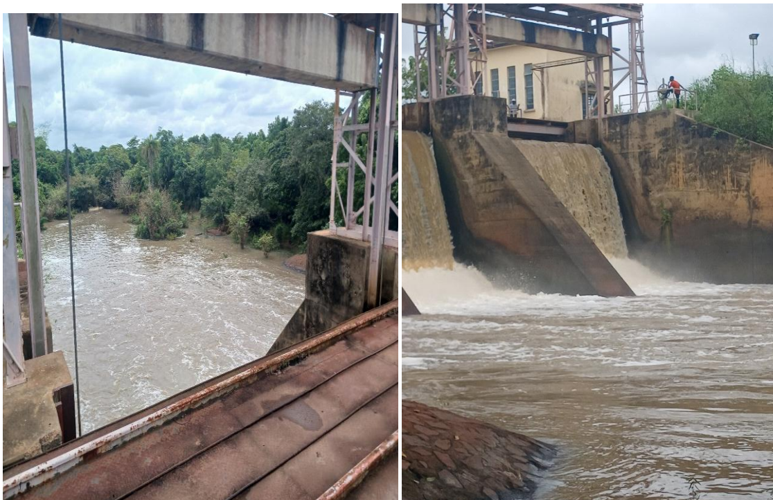
Figure 3.6b: Another view of the dam from the Water Corporation side
