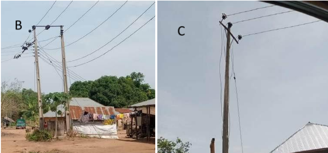
Plate 4.18b and c: Social infrastructures at Ijaiye A – abandoned borehole, B - electric cables and wires without a transformer, and C – fallen poles
